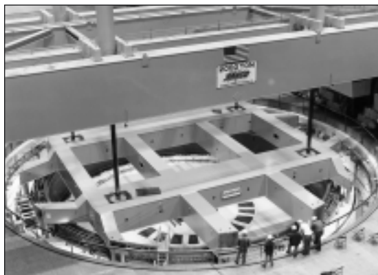
Photo 2. Refurbished stator of Grand Coulee unit G-24 being lowered into the pit.
