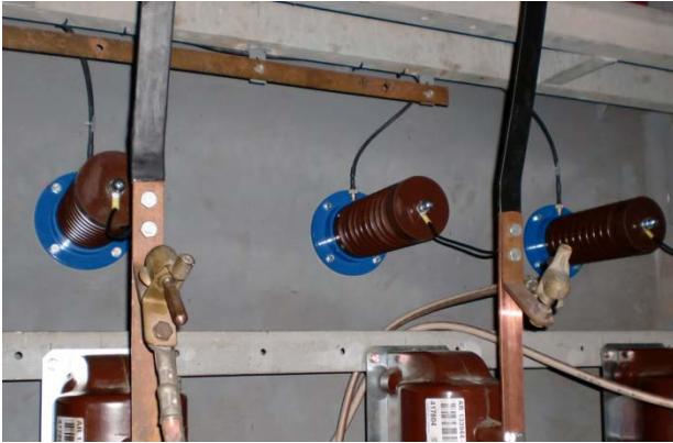
Figure 4 Capacitive sensors installed horizontally
