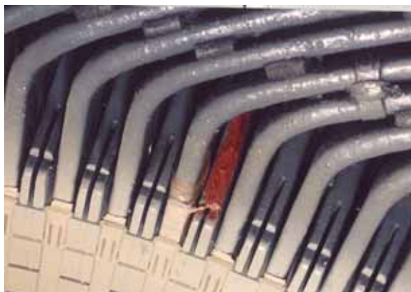
Fig. 2. Stator slot coupler installed under wedge in 160 MVA machine
