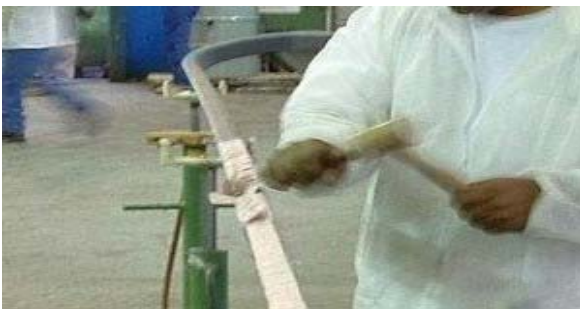
Fig. 10 Stripping of ground insulation in preparation for reinsulation of the stator bar. This is a method of quickly returning the failed or damaged bars back to service if spare bars are not available. This method is not possible if bars are severely damaged.
