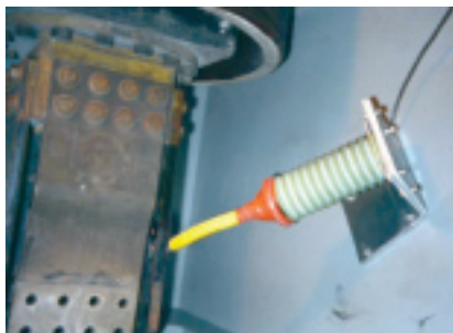
2. Partial-discharge sensor can provide considerable information on generator condition
