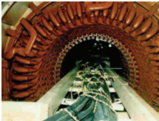
24. Excitation coil is arranged for high-flux test
