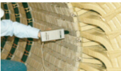
21. Hand-held taper checks tightness of stator wedges
