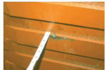
14. Significant core damage above could be overlooked by the untrained eye
