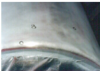
25. Minor indications are highlighted on the retaining ring after NDE
