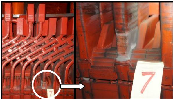
Fig. 30 PD on Cirata Unit 7 slot no.7
