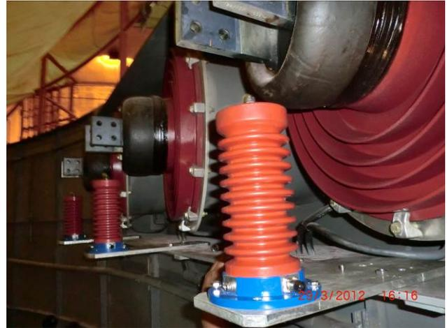
Fig. 4 PD Sensors installed at generator terminals
