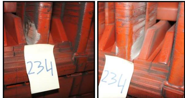
Fig. 34 PD on Cirata Unit 7 slot no.234 (both on left side and right side)
