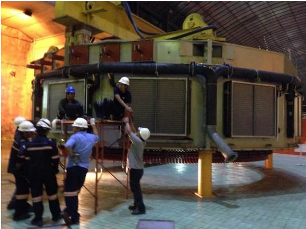
Fig. 29 Stator PLTA Cirata Unit 7 after pull-out
