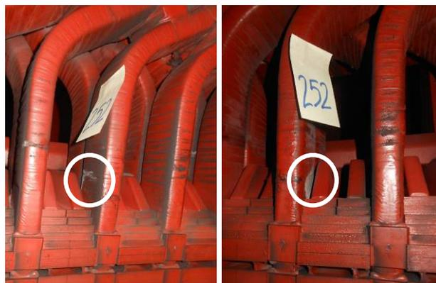
Fig. 35 PD on Cirata Unit 7 slot no.252 (both on left side and right side)
