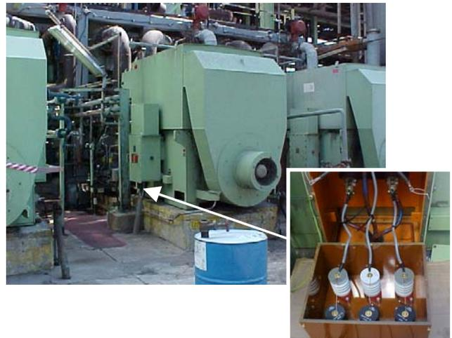
Fig. 8 Motor and temporary coupler connection.
