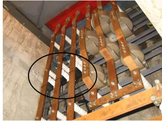
Fig. 4 Temporary couplers mounted on the compressor bus-bars.
