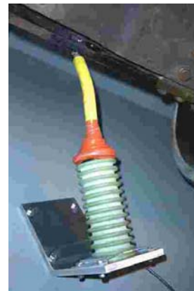
Photo 1. Iris Power Engineering Capacitor
