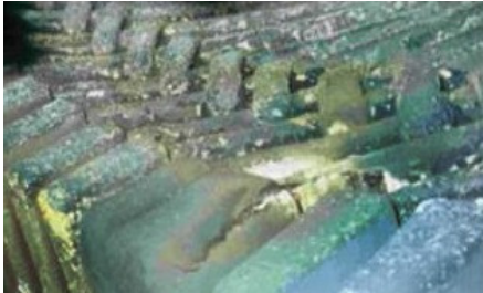
11, 12. Inadequate clearances at phase-to-phase locations difficult to insulate are conducive to failed connections (left). At right is copper burning caused by a non-mica connection insulation failure
