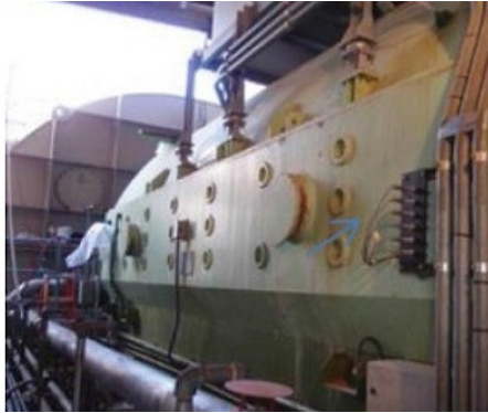
9, 10. Core-to-frame support structure at left is for the generator at right. Welded method of attachment without vibration isolators increases the susceptibility of the generator to frame and foundation cracking
