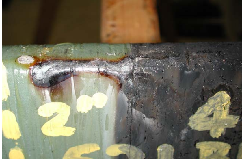
Figure 2 Insulation failure of a stator coil in the voltage endurance test at 283 hours.
