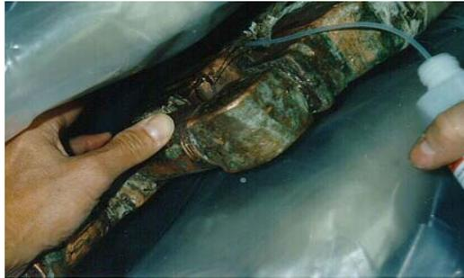
**Figure 31. Testing for Water Leak using Bubble Solution**
