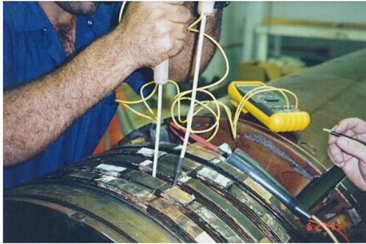
**Figure 16. Checking Pole/Coil Voltages with Retaining Ring Removed**
