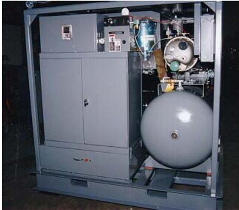
**Figure 26. Test Skid for Removing and Drying Water from Stator Windings (General Electric)**
