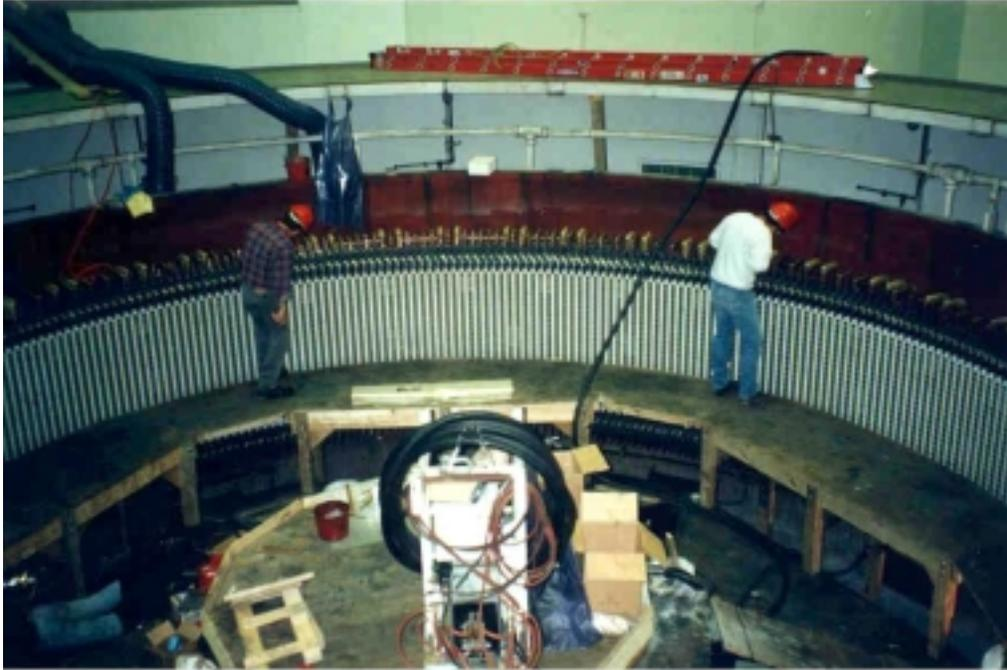
Figure 1: Installation of Partial Discharge Sensors in a Hydrogenerator
